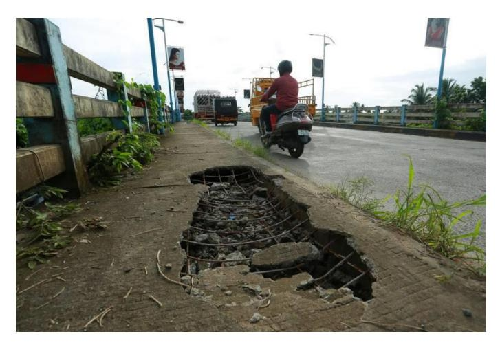
A broken footpath on the bridge on the mini bypass road in Thripunithura across the Thattappallikkattupuzha in Kerala, posing grave danger to pedestrians in June 2022. Photo: R.K. Nithin/The Hindu
